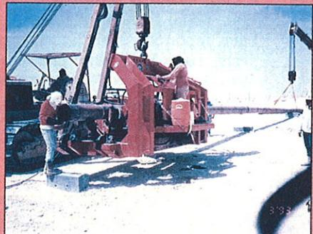
**The field joining unit can be suspended by a sideboom tractor and easily moved down the pipeline.**
